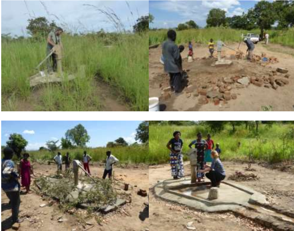
Figure 5. Before and after civil work improvement at 4. Manoro
