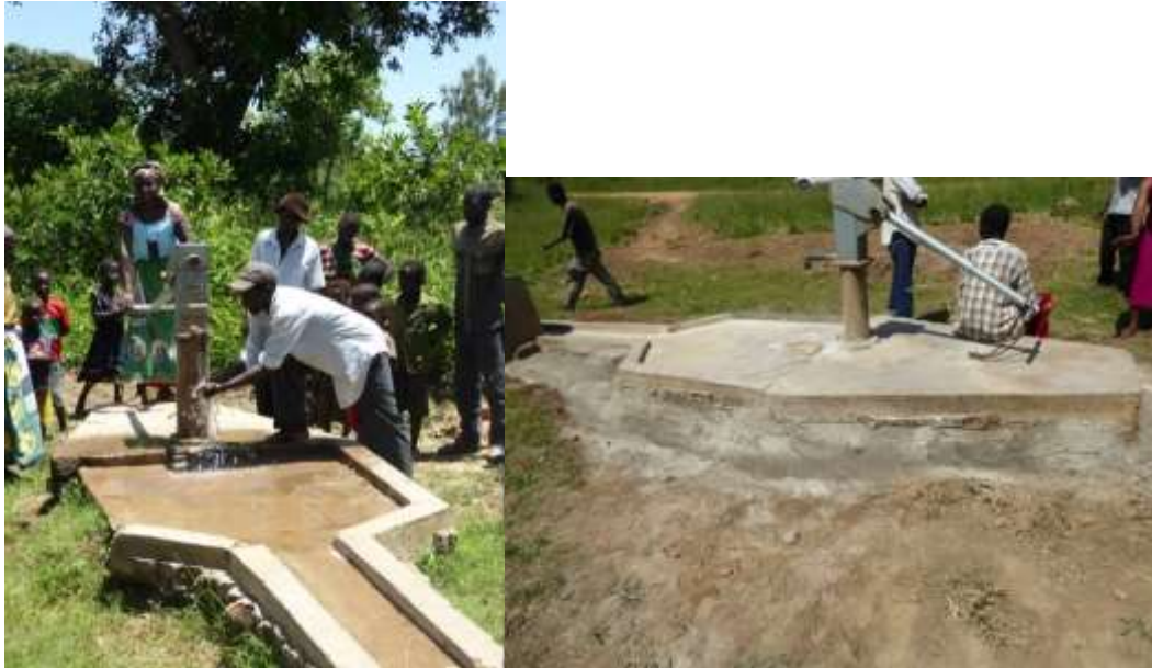
Figure 4. Before and after civil work improvement at 5. Kalanga.
