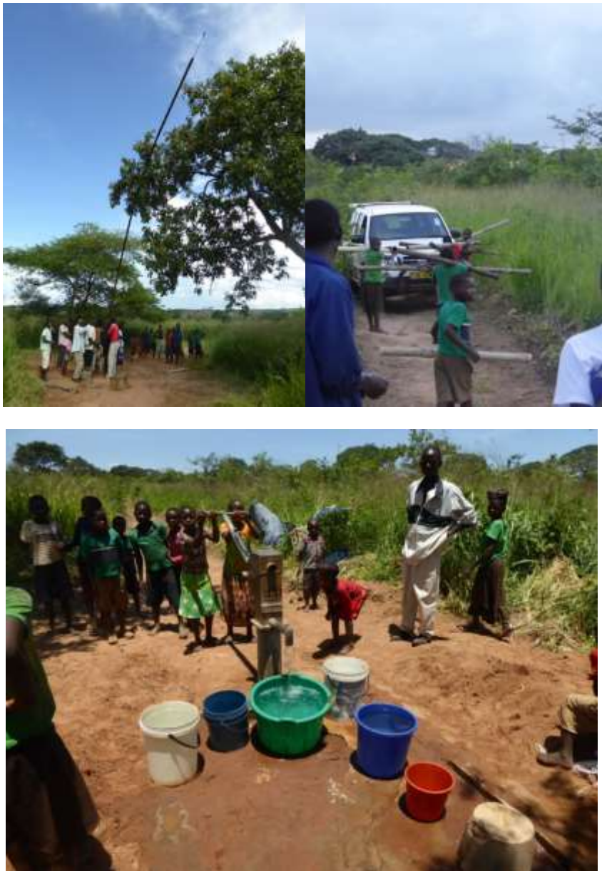
Figure 7. Rehabilitation at 8. Manoro
